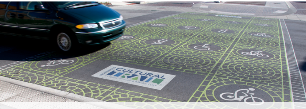
Using distinctive pavement materials like painted concrete can help slow traffic and encourage drivers, pedestrians and cyclists to better identify where and when pedestrians may be crossing.
